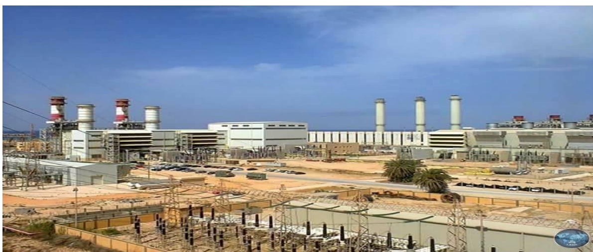
Figure 3. Benghazi combined cycle power plant
